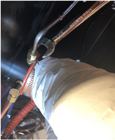
Install Compression Fitting and TC
